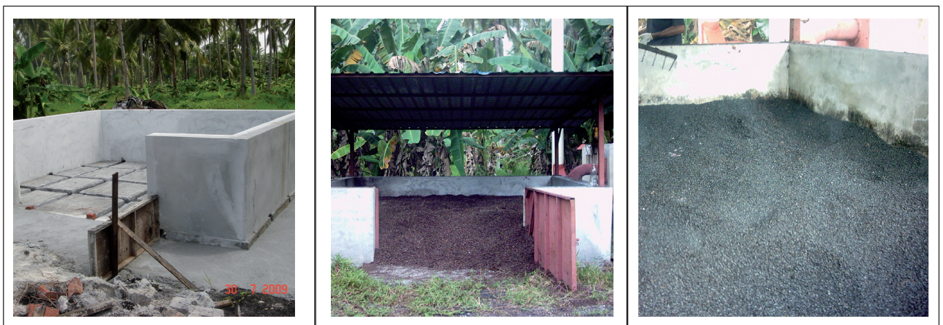
(a) Building the system
