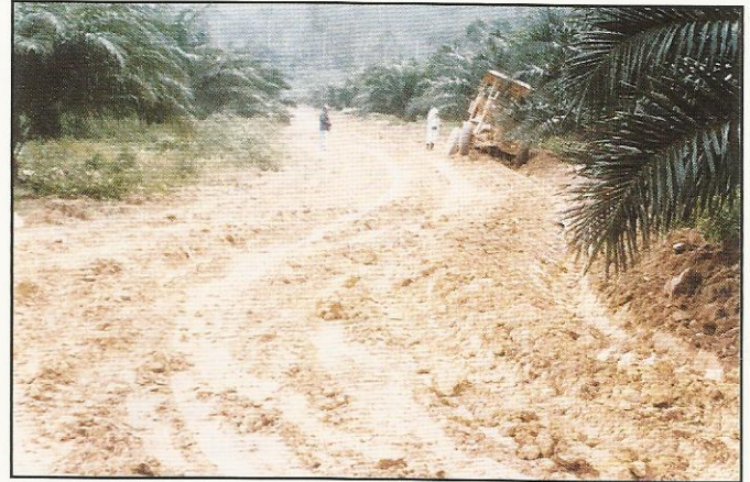
Plate 2. Surface leveling and side drain construction
