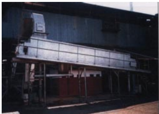
Figure 6. Continuous sterilization pilot plant
