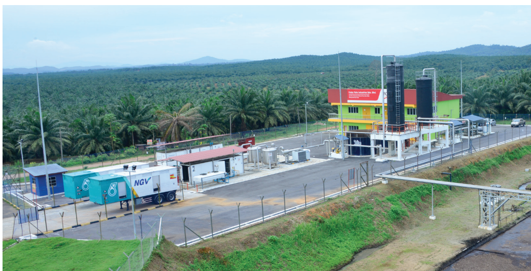
Figure 1. The 400 m 3 hr -1 Bio-CNG commercial plant at Sg Tenggi Palm Oil Mill.
