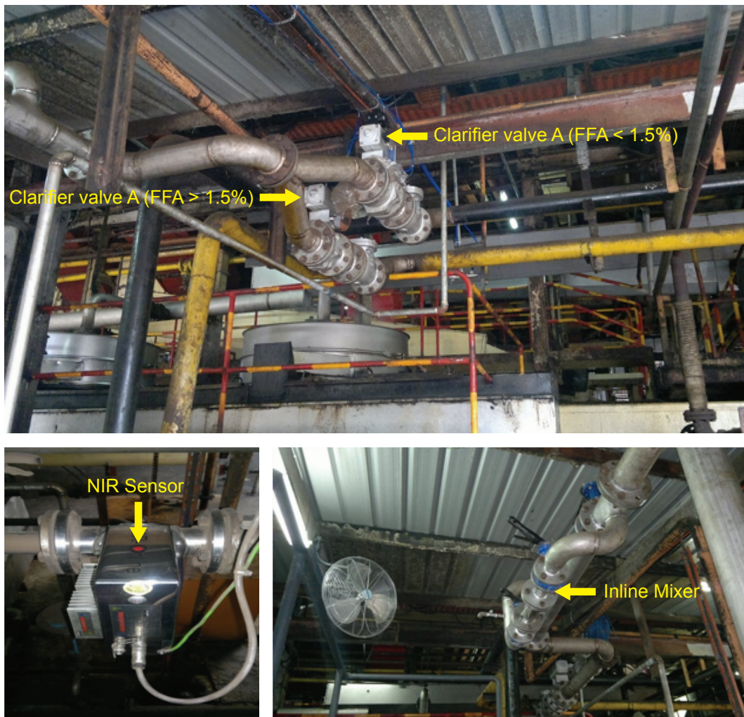
Figure 3. NIR Online system in the mill.
