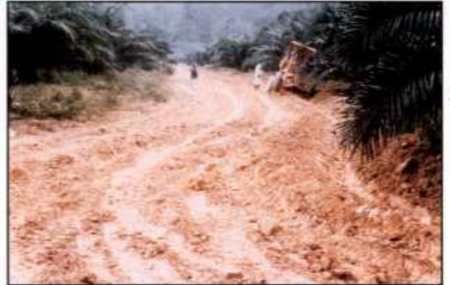
Plate 2. Surface leveling and side drain construction
