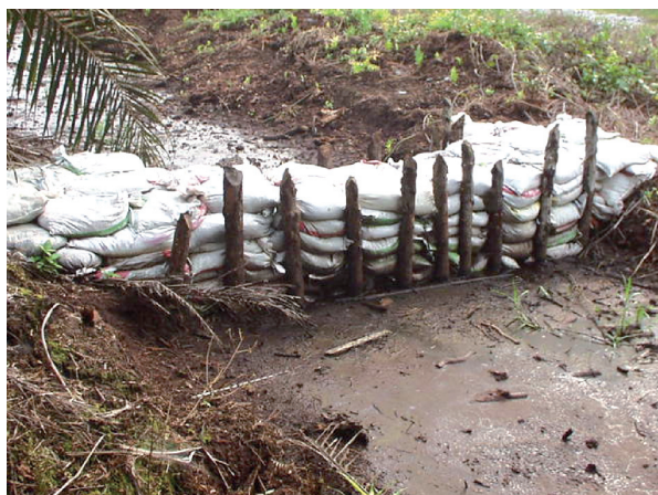
Figure 2. Adjustable weirs made from sandbags.
