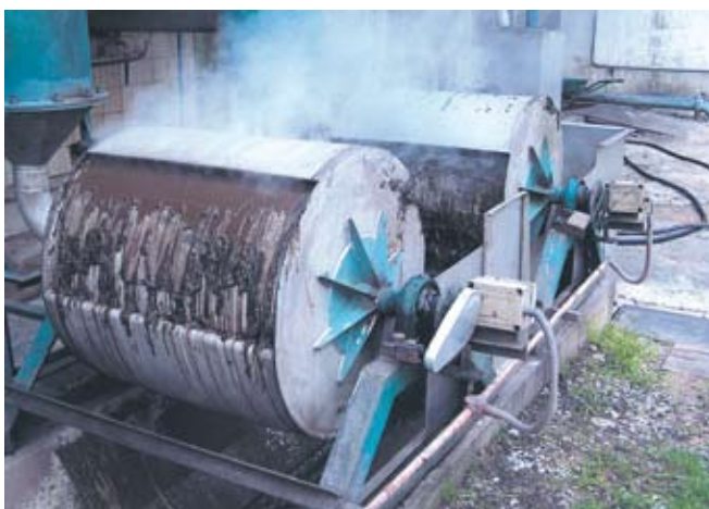
Figure 1. Sludge measured by rotary basculator.
