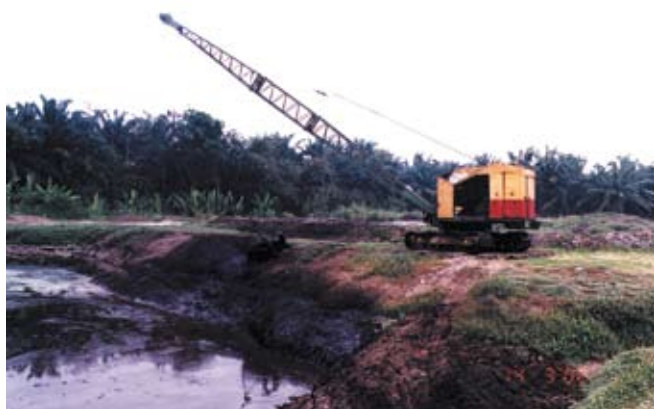
Figure 1. Conventional pond cleaning by excavator.
