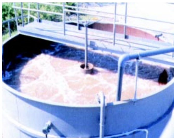
Figure 3. Top View of Reactor Showing Effective Aeration.
