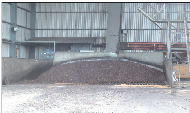
Figure 1. Loading ramp for palm kernel at a kernel crushing plant.
