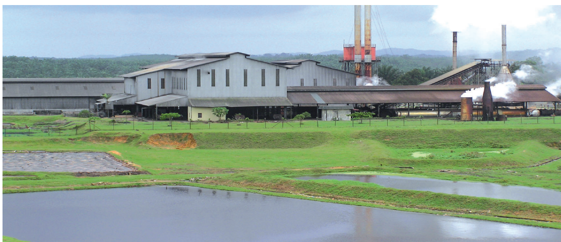
Figure 1. A typical palm oil mill with an effluent pond.
