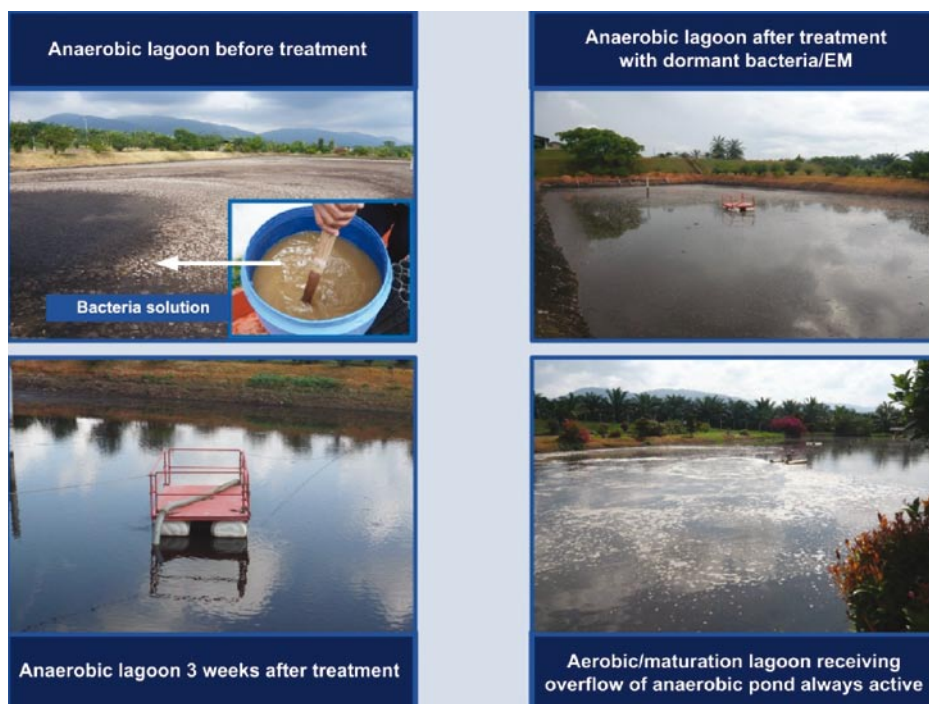
Figure 1. Application of dormant bacteria to the anaerobic lagoon of a palm oil mill.
